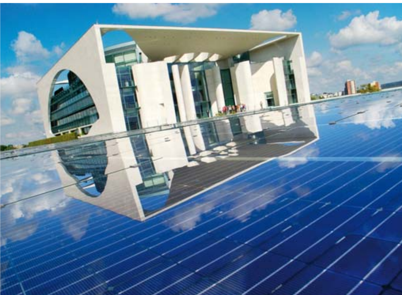
150 KW capacity photovoltaic facility on the roof of the Bundeskanzleramt (Federal Chancellery), Berlin, Germany ©Paul Langrock/Zenit/Greenpeace
