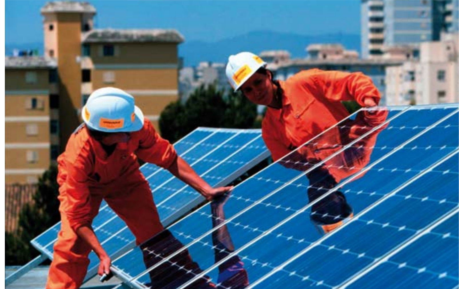
Installing solar panels on a school in Spain. A DE strategy has the potential to create jobs as well as encouraging technological development. © Greenpeace/Shirley
