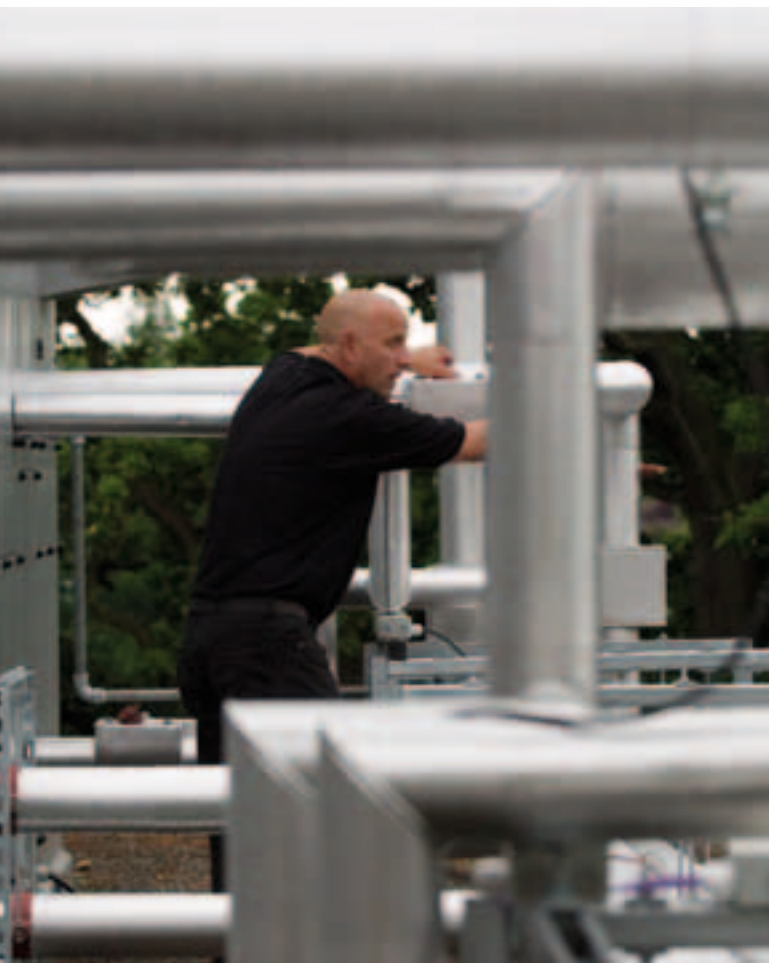
Air conditioning on the roof of Woking's leisure centre, powered by a trigeneration plant that offers cooling for extra emission savings. ©Greenpeace/Cobbing.
