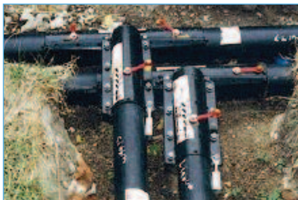
Figure 2: Pre-insulated heating flow and return pipe work within a trench
