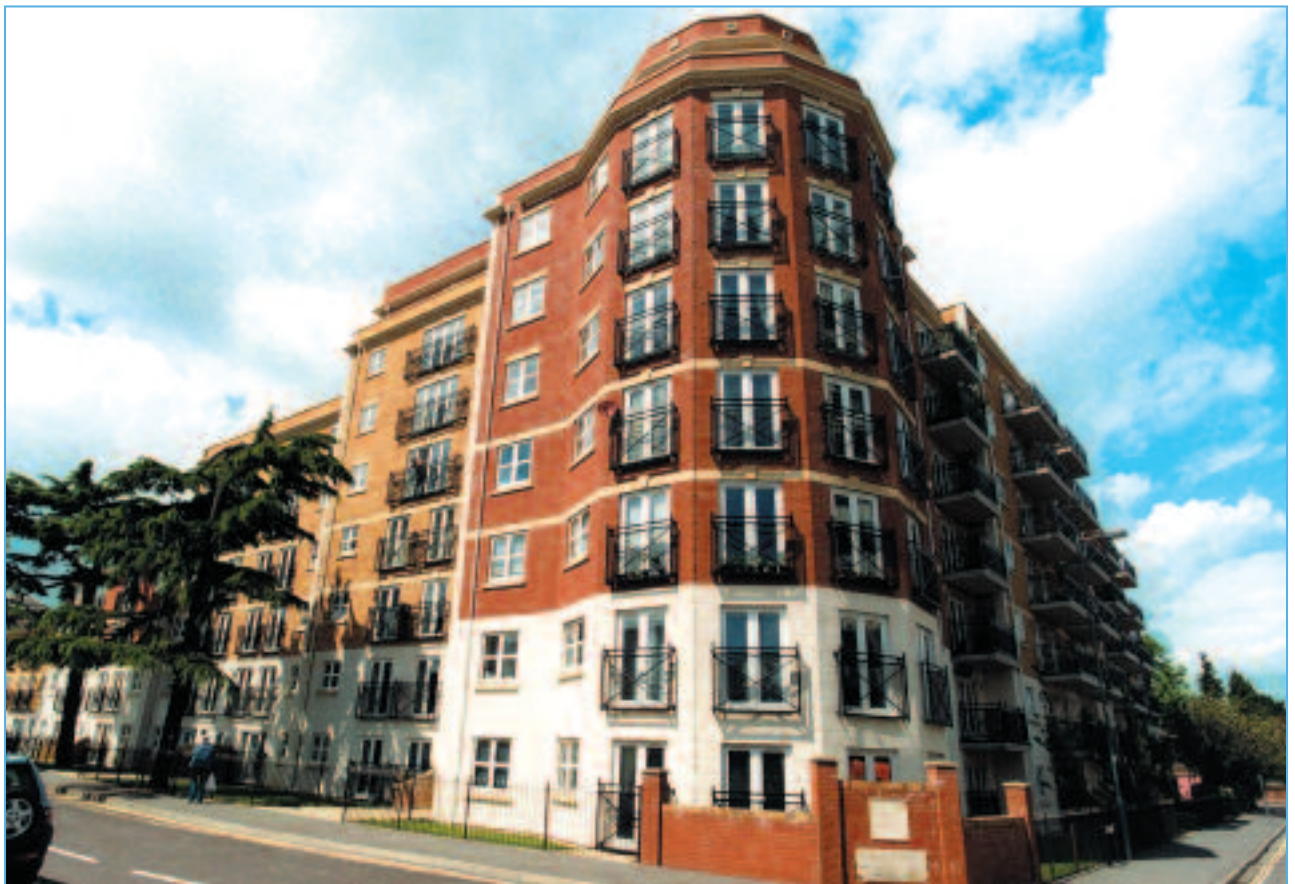
Figure 6: Park View – a new residential housing block connected to community heating
