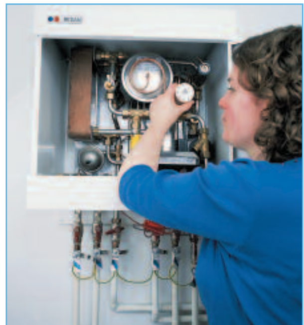
Figure 3: A typical hydraulic interface unit (HIU)
