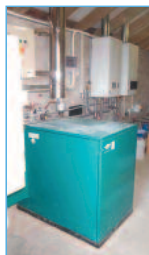
Figure 9: Station Road, Newmachar, Scotland, with energy centre building in foreground and the 5.5kWe CHP unit and two wall-hung gas condensing boilers.
