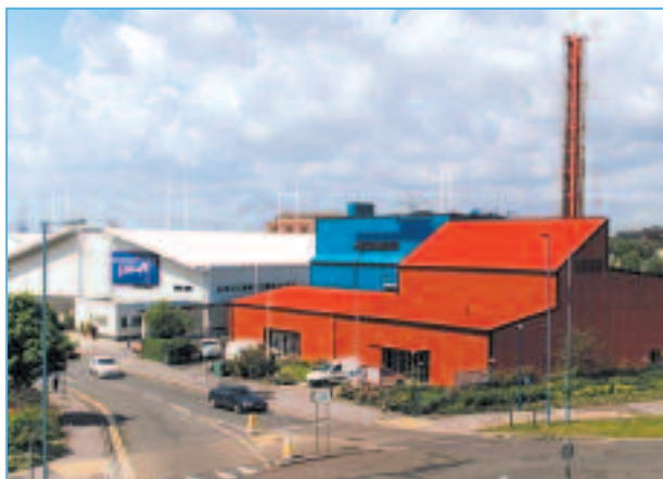
Figure 7: The Southampton Energy Centre
